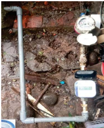
Figure 3: Smart meter installed along with existing meter (Source: DBD Water Systems)
